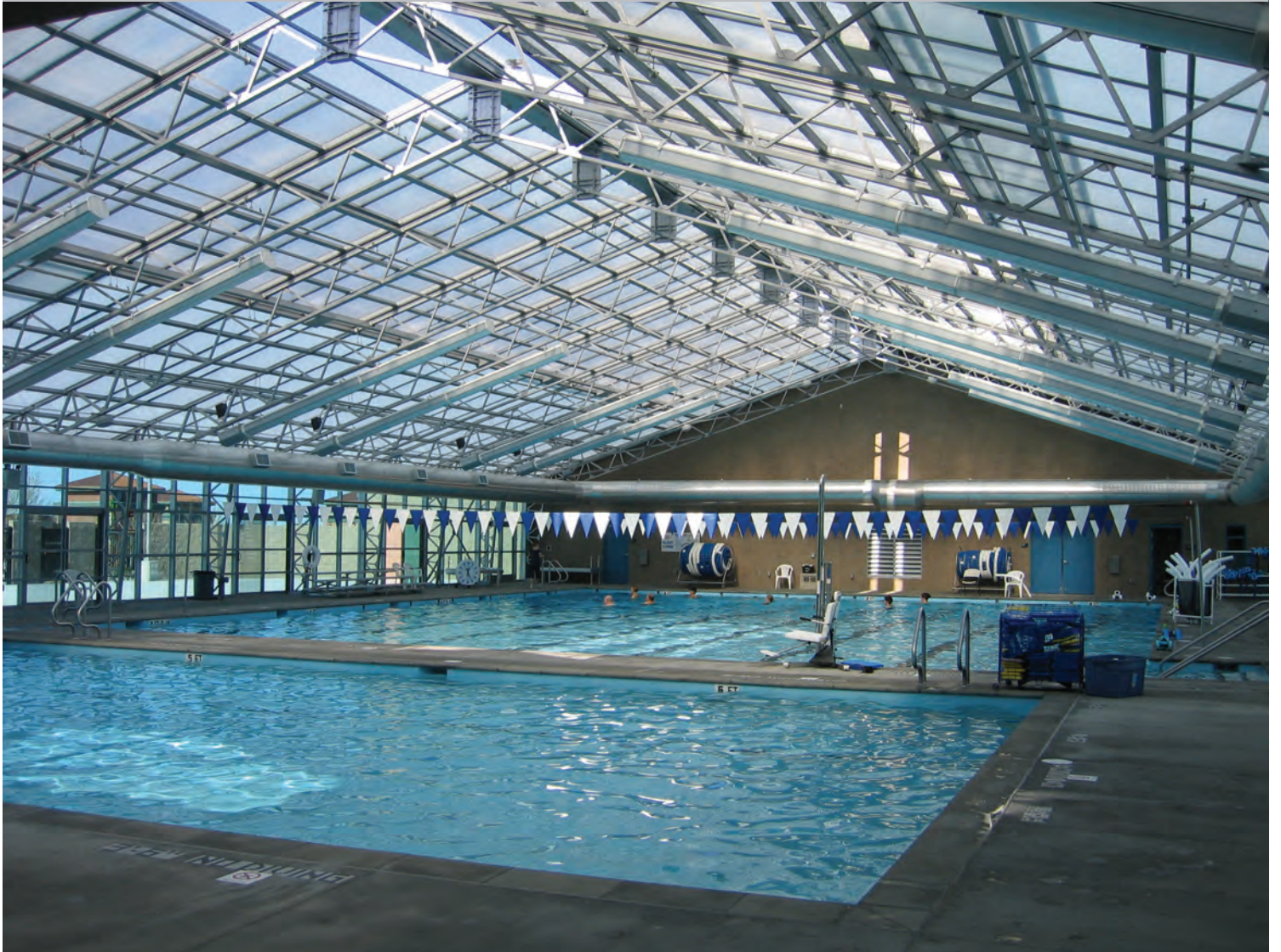
City of Roseville's Mike Shellito Indoor Pool.
